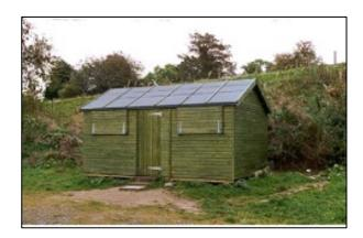
Basic fishing hut. Timber weatherboard construction with felt roof and timber floor. No services.
