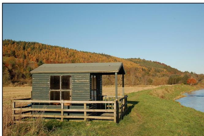
Simple fishing hut. Timber weatherboard construction with felt roof and timber floor. No services.
