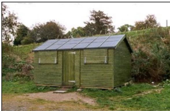
Basic fishing hut. Timber weatherboard construction with felt roof and timber floor. No services.
