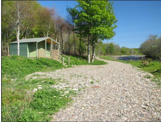
Fishing hut of timber weatherboard construction with profile steel sheeted roof.
