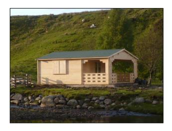
Fishing lodge constructed of pre-formed 125mm (5") logs, erected on a concrete floor slab with slate roof.
