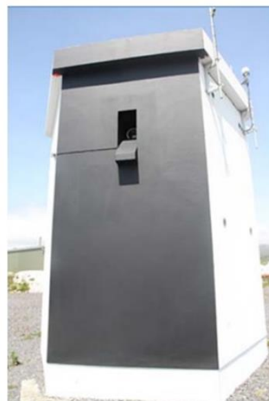
Example of Direction Light & blockhouse with PEL installed internally.
