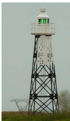
Example of basic lattice structure (approx. 15m tall)
