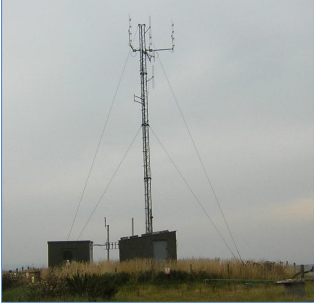
Local Area Broadcast Mast
